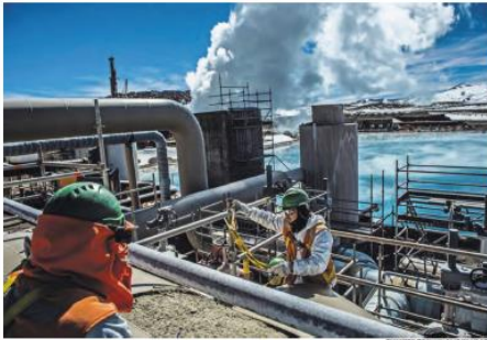
Workers installing pole foundations at South America's first geothermal energy plant, located in Cerro Chibola, Chile. The new plant will be able to power about 100,000 homes.
