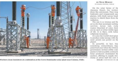
Workers clean insulators at a substation at the Cerros Dominador solar plant near Calama, Chile.
